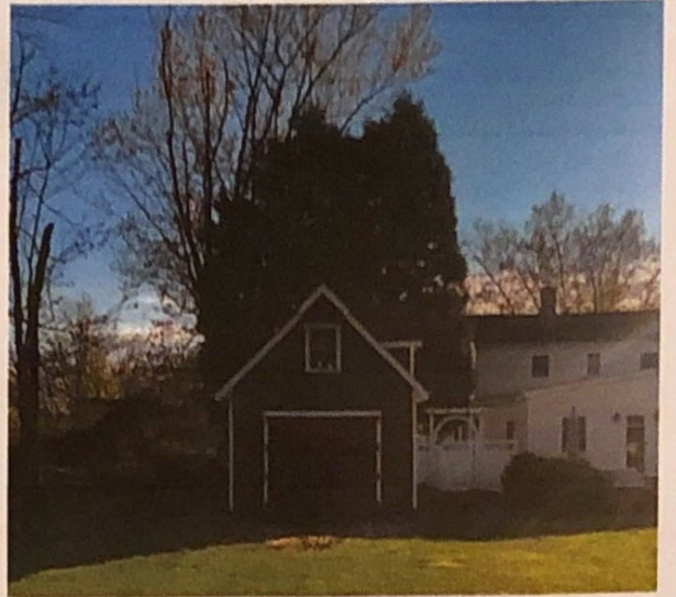
View from Back Yard 2
