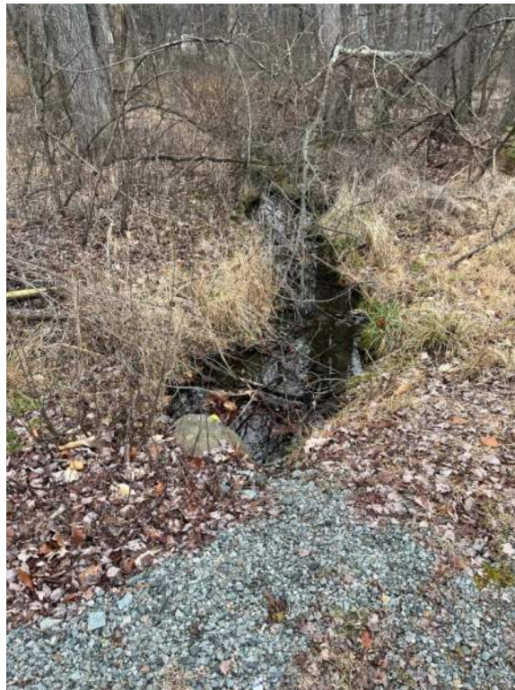
Stream at 12" Diameter Pipe Outfall at Northwest Portion of Property
