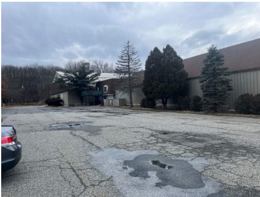
Existing Building with Adjacent Trees
