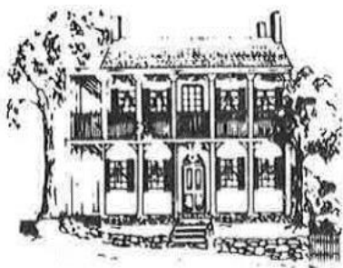
Phoenix House c. 1820
