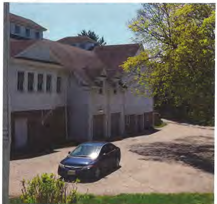
Outbuildings at Hilltop Road Entrance
