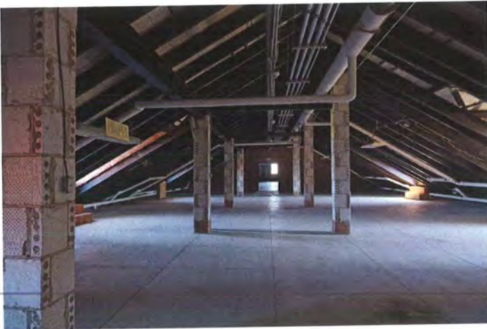
Attic space to be converted to units
