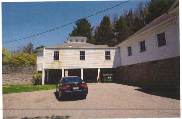
Outbuildings to be rehabilitated and converted into affordable housing units
