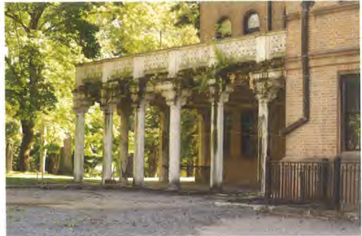
Covered porch to be restored Image taken by HLW
