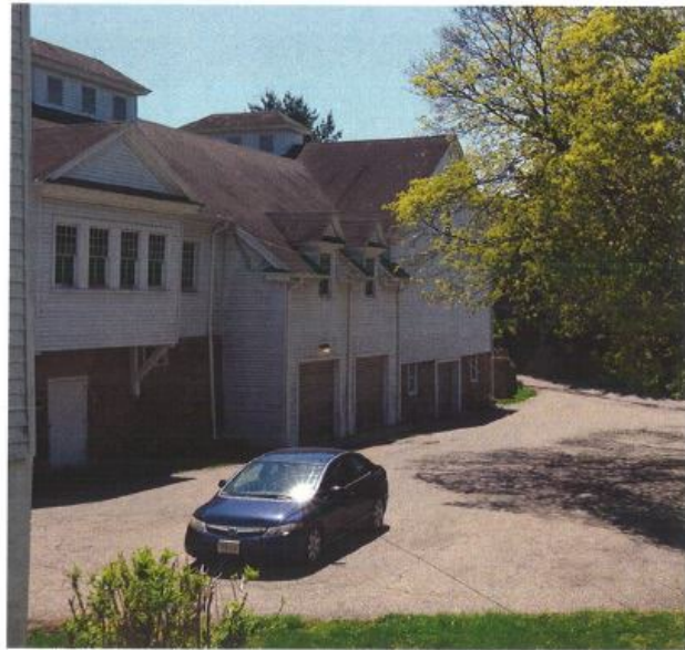
Outbuildings at Hilltop Road Entrance
