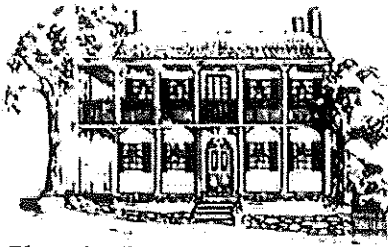
Phoenix House c. 1820
