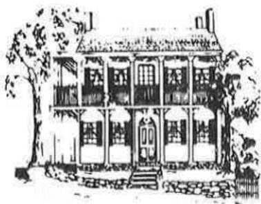
Phoenix House c. 1820
