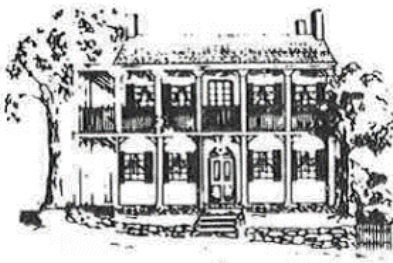
Phoenix House c. 1820
