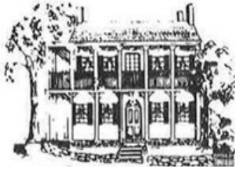
Phoenix House c. 1820
