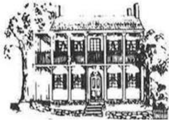
Phoenix House c. 1820
