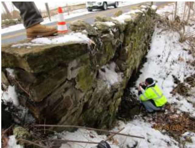
Engineers Examining the Bridge Structure
