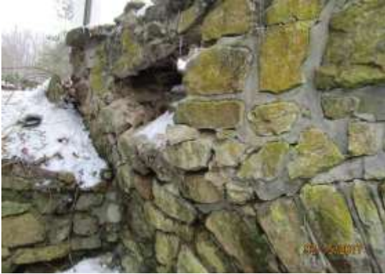
Side view of Hardscrabble Road bridge
