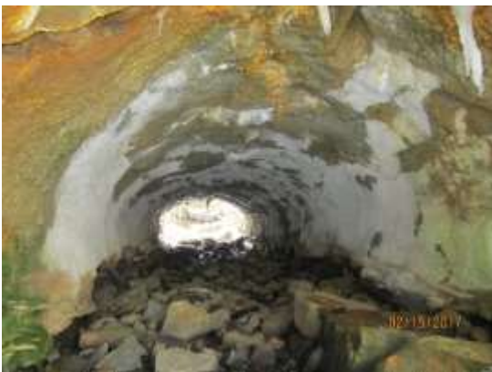
Underside of Hardscrabble Road bridge
