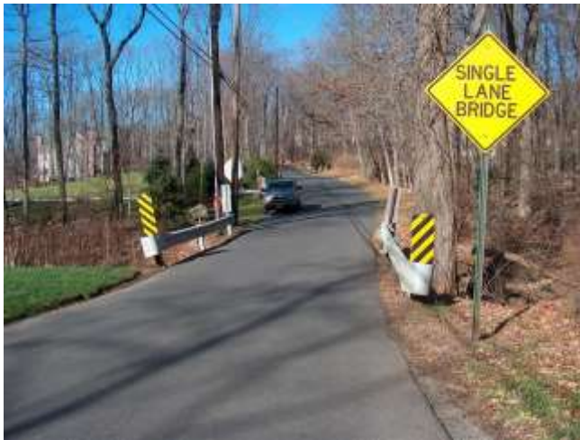
Combs Hollow Road bridge
